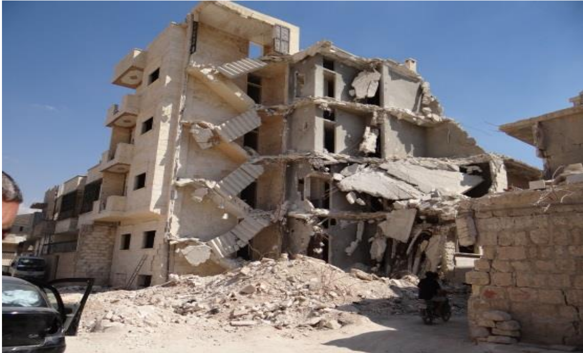
Housing destroyed in Marafat Numan – 20 people were killed in this building
