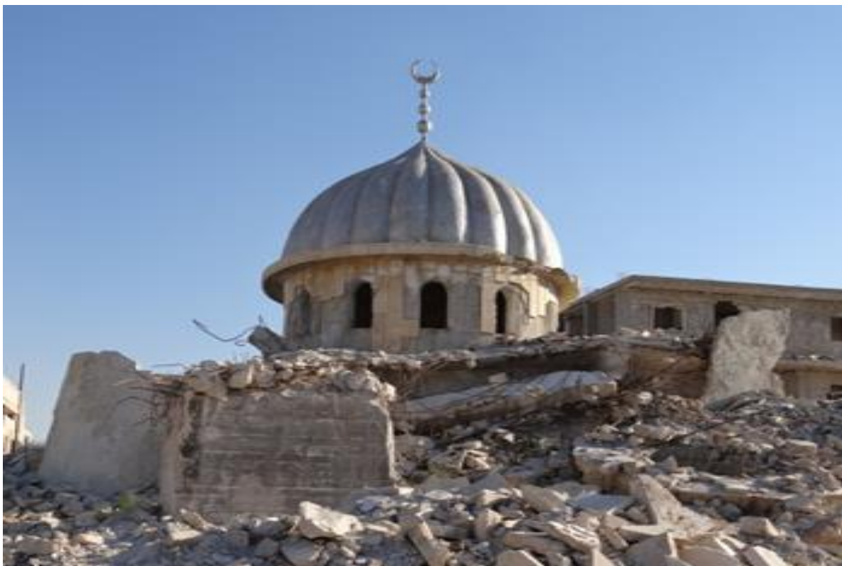
Masjid completely destroyed
